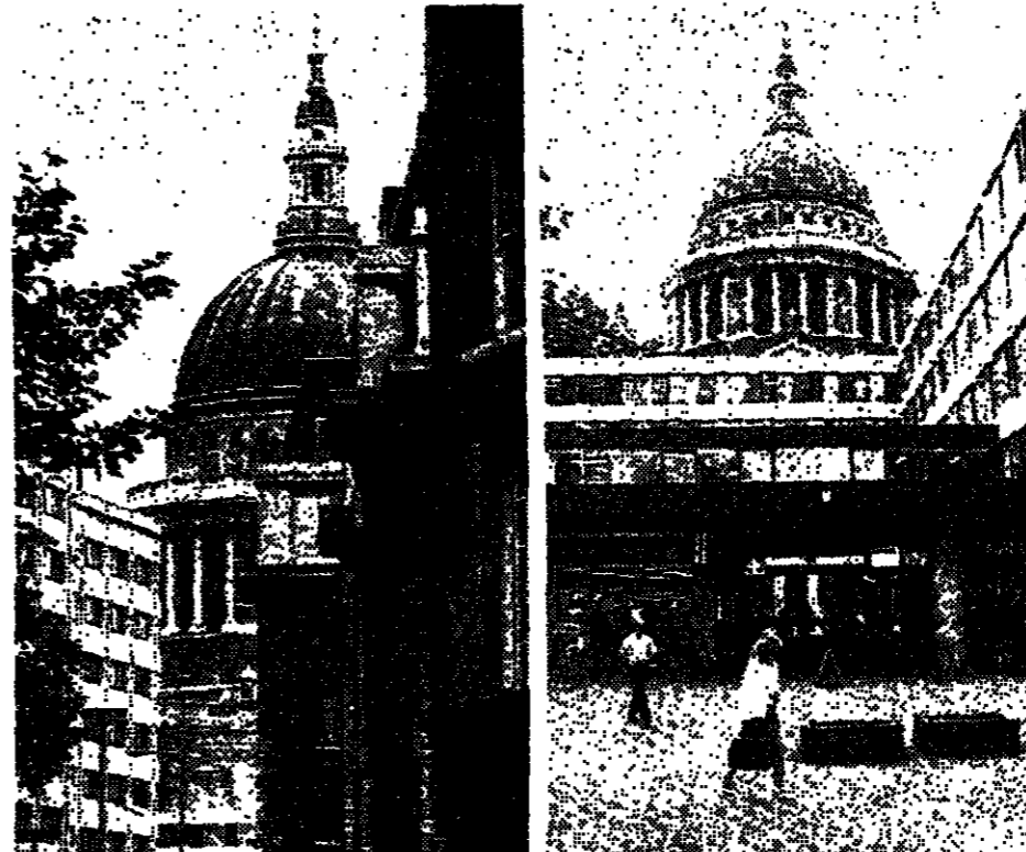
A promising view from the north side of the Cathedral from Bartholomew Close near Bart's Hospital (left) and through the sixties "brutalism" of Paternoster Square, whose developers at least kept the Wren masterpiece in sight (Photographs: Graham Wood).
